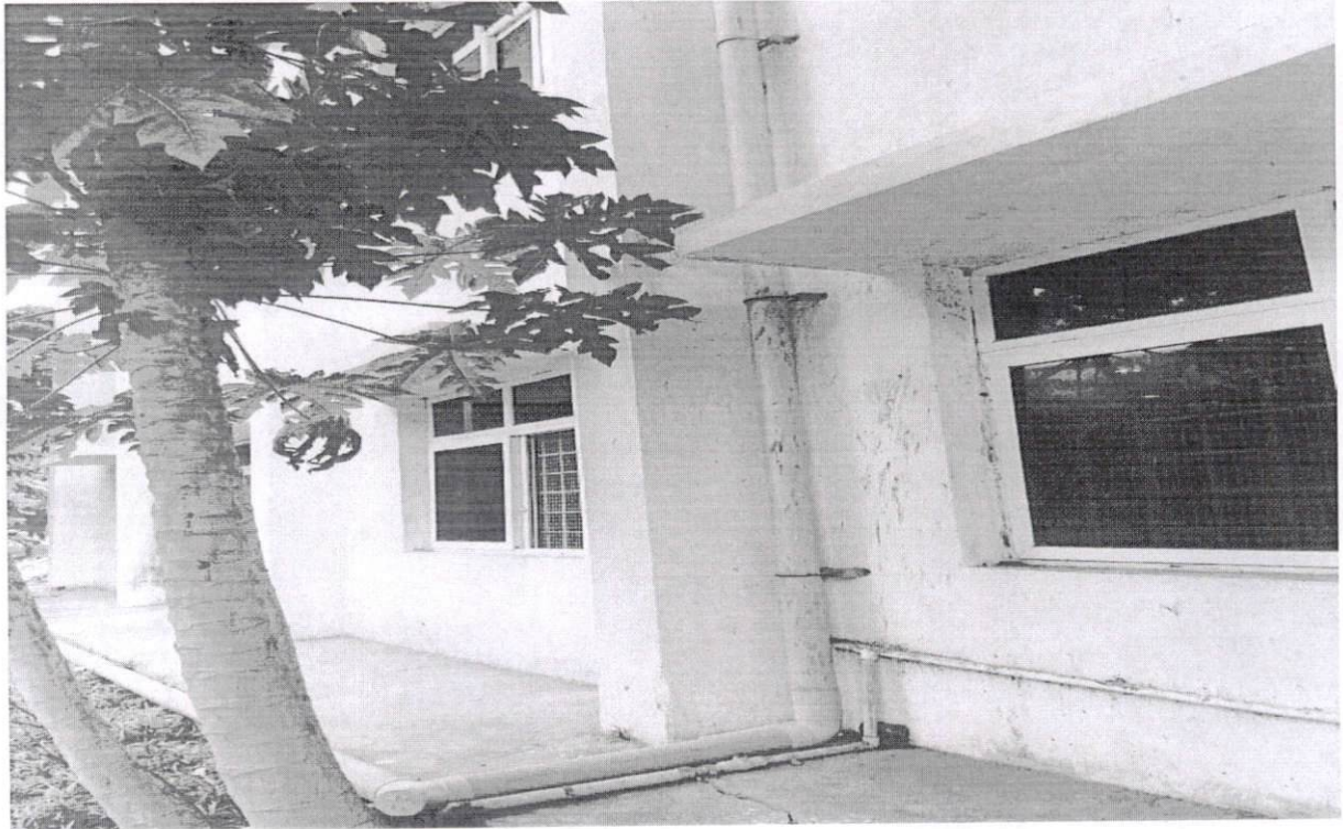
Geotagged photo of pipe distribution from overhead tank to rain water storage
