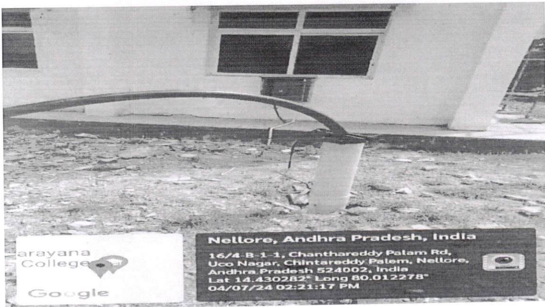
Geotagged photo of pipe distribution from overhead tank to rain water storage
